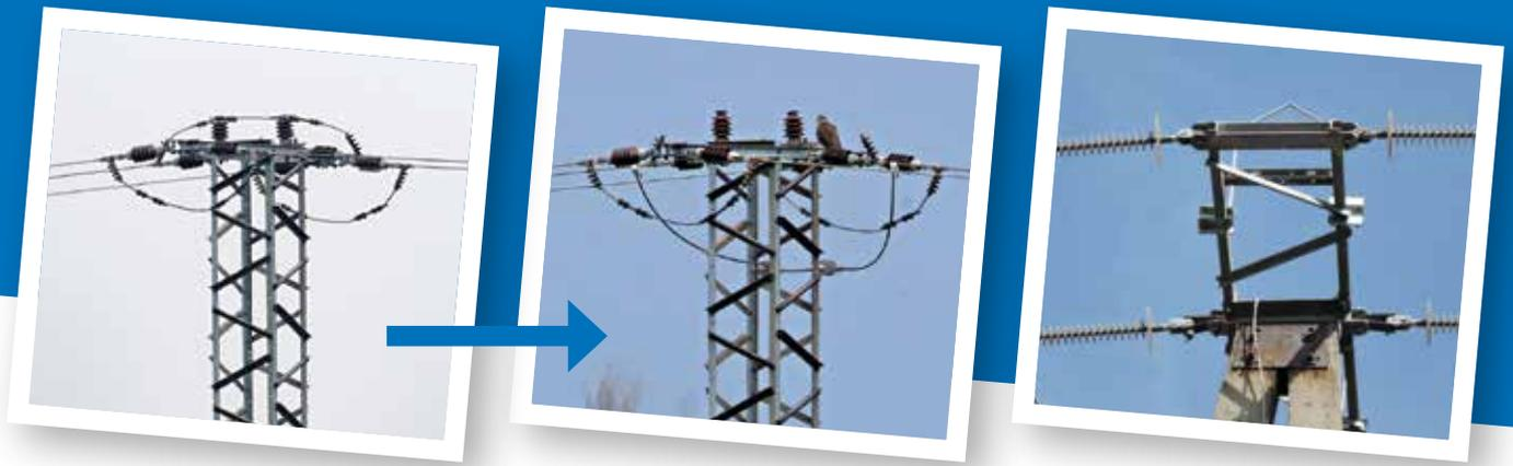
Even the riskiest poles can be made more safe by only changing one exposed jumper wire for the suspended type. It is a simple, effective, and cheap solution applied on 22 kV poles in Slovakia. Bare wires are replaced with insulated ones, the mortality rate has been reduced to zero. Also in case of changing the insulator to the 800mm long new type, and using insulated power connections, the mortality could be eliminated from the most dangerous type, the tension poles.
