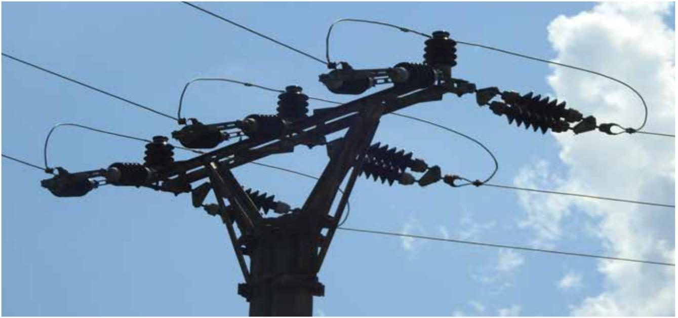
The risk of electrocution for a bird mainly depends on the design, and configuration of the pole. Certain types, especially metal structures with a horizontal location of cross-arm and jumper wires (e.g., top over the cross-arm) and pin insulators, are among the riskiest. It can be said that the more complex the structure and the shorter the distances between the parts of the structure, the risk also for smaller bird species increases.
