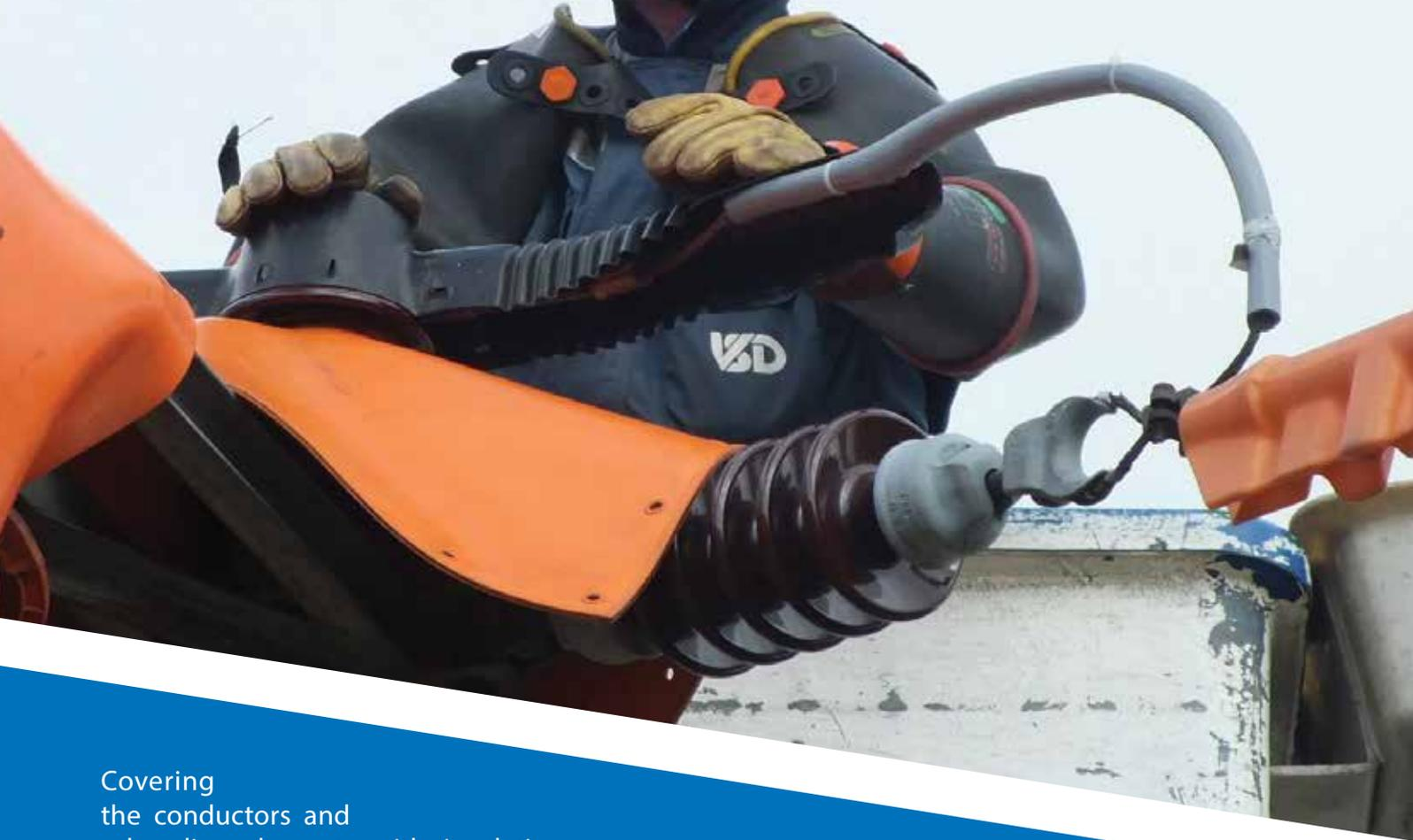
Covering the conductors and other live elements with insulating materials can help to reduce the mortality risk and can be also effective solution. This solution is the very common, universal and is used in many countries and by many grid operators. On metal cross-arms, another possible type of insulation consists of placing rigid plastic covers on the parts where birds perch, so that they avoid contact with the ground connection of the pole.
